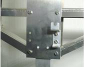
brackets have been positioned, tighten the nuts and bolts.
