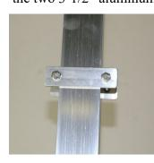
the two 3-1/2" aluminum plates to the pole using two 1/4" x 2-3/4" bolts with flange nuts. The stop should be mounted above the hub and adjusted according to the height of your martin house.
